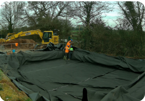
Installation of impermeable membrane.
