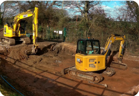
Excavation of shallow basin.
