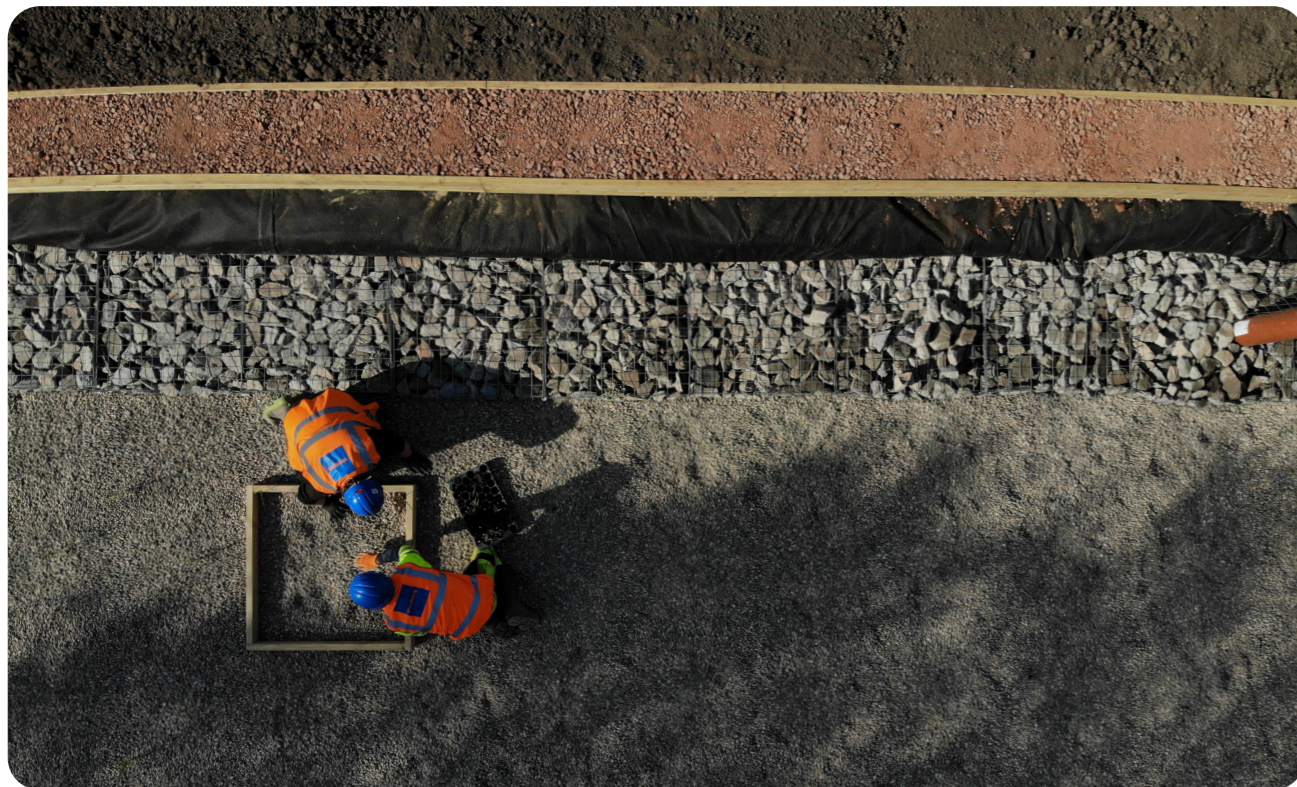
Planting of reeds into top layer of fine gravel.
