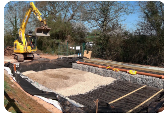
Installation of first layer - coarse gravel.
