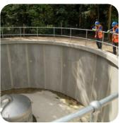
contaminants and turbidity. Contaminants and sediments were filtered through silt tanks prior to discharge to eliminate the risk of pollution.
