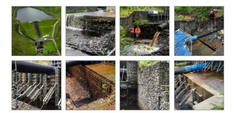
Stonbury was contracted to deliver repairs to a spillway in Lancashire after the existing gabion baskets supporting the structure had degraded.
