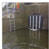
Flap valves are important to prevent reverse flow of water into holding structures, protecting water assets from contamination, animal ingress and flooding. The Drinking Water Inspectorate (DWI) recommends that flap valves should be installed on drainage and overflow routes and inspected every six months.
