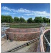
Stonbury completed masonry repairs to three bio-filter beds in the South of England. The works took place in sequence to allow the bio-filters to remain in service for the twenty-week construction program duration.
