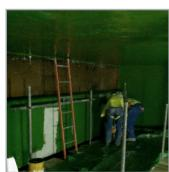
Following a non-destructive testing (NDT) survey at a WWTW, it was identified that major concrete repairs were required to five tanks, to ensure the plant could remain in use. However, the works could only be undertaken during a full plant closure.
