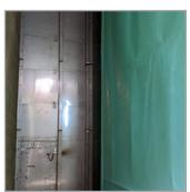
Stonbury was contracted to produce and install a new solution to increase the water quality output from two Water Treatment Works contact tanks, after the client's recent step tests highlighted that at flows exceeding 20MI/d, output failed to meet the minimum disinfection contact requirement.
