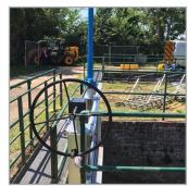
Following a successful tender, Stonbury was engaged by a client to design a trash screen that incorporated a manually operated vertical penstock screen. Once the design was approved, the screens were manufactured and installed to three sluices located on a weir structure. The works required a Flood Risk Activity Permit (FRAP), which was obtained from the Environment Agency (EA).
