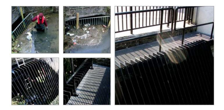
Stonbury was asked by North Somerset Council to design, fabricate and install a new trash screen at an underground river culvert in Clevedon, Somerset.
