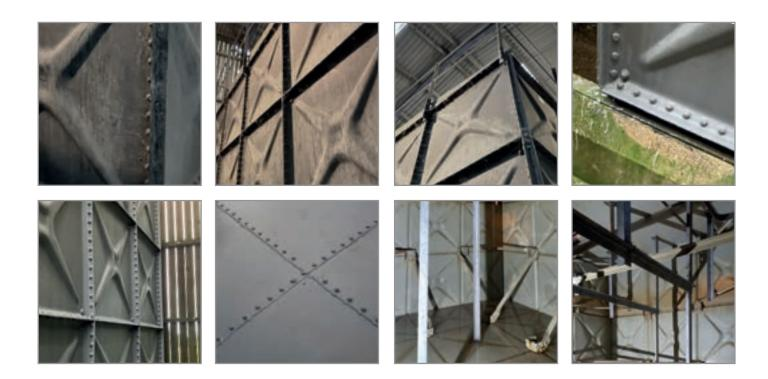
Refurbishments were required on the 0.9 trillion-cubic-metre tank due to degradation of the side panels and instability of the roof. The refurbishments, which have eliminated the requirement for a new tank, have increased the lifespan of the asset by twenty years, saving Stonbury's client over two million pounds.
