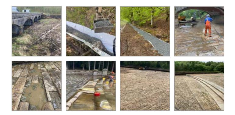
As part of a large multi impounding reservoir spillways programme, Stonbury was contracted to complete works to a historic spillway and head wall as part of both safety and maintenance requirements.
