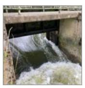
Early contractor involvement resulted in a timely and cost-effective solution for a seized sluice gate that was causing uncontrolled flows.
