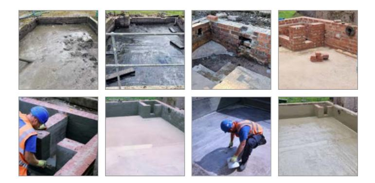
As part of a significant multi-site wastewater treatment works framework, Stonbury was pleased to deliver the refurbishment of a brick sludge tank, returning the vital asset back to service.
