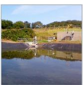
To extend the life of two final settlement lagoons, Stonbury was required to carry out refurbishment works, which included repairs to the outfall structure, the installation of an EPDM liners and replacement pipework.
