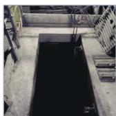
Due to severe hydrogen sulphide attack, Stonbury were contracted to rebuild a failing inlet chamber at a wastewater treatment works (WWTW), this included the replacement of all defective rebars within the walls.
