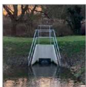
Stonbury has been contracted by the Environment Agency to replace the headwalls on a storm water drainage pipe in an embankment that had become destabilised by natural erosion.
