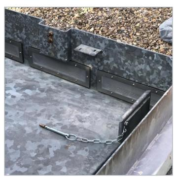
As part of an extensive refurbishment programme, Stonbury have been replacing the push-fit vents used inside security access covers on reservoir roofs. The vents allow air to pass through the reservoir while preventing insects, small animals and debris from entering the tank.
