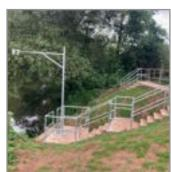
Stonbury was contracted to design, manufacture and install a bespoke two-headed, pole-mounted radar bracket to measure water height levels at a gauging station in the midlands.
