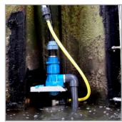
Stonbury were asked to investigate the use of hydraulic ram pumps as an alternative to electrically powered pumps for the Environment Agency, who required the installation of an eel pass on a crump weir in Bristol.
