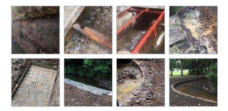
A county council contracted Stonbury, to carry out a package of repair works to dams and watercourse at various locations. The repairs were required due to deterioration of the masonry, erosion, tree root damage and water ingress.
