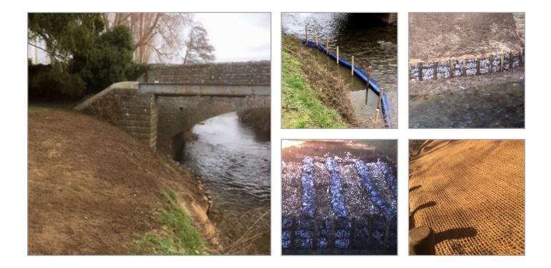
Stonbury were contracted to carry out comprehensive restoration works to a failing river bank that had become very unstable due to a water main leak.
