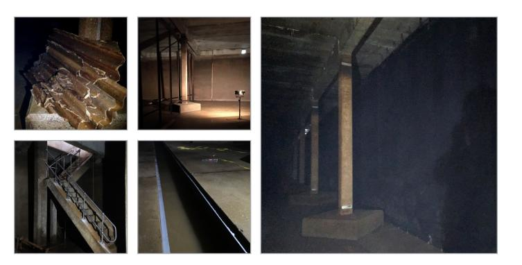
Due to the presence of Chrysolite Asbestos inside a drinking water contact tank, Stonbury were contracted to remove a contaminated baffle wall and it's supporting steel structure. The wall was to be replaced with a new thermoplastic baffle curtain.
