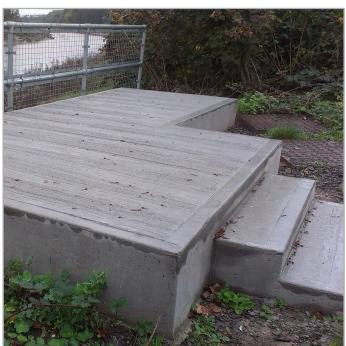
Stonbury was asked to fabricate and install a bespoke access gantry, fencing, ladder and gate at an outfall in Bristol due to unsafe access for maintenance teams.
