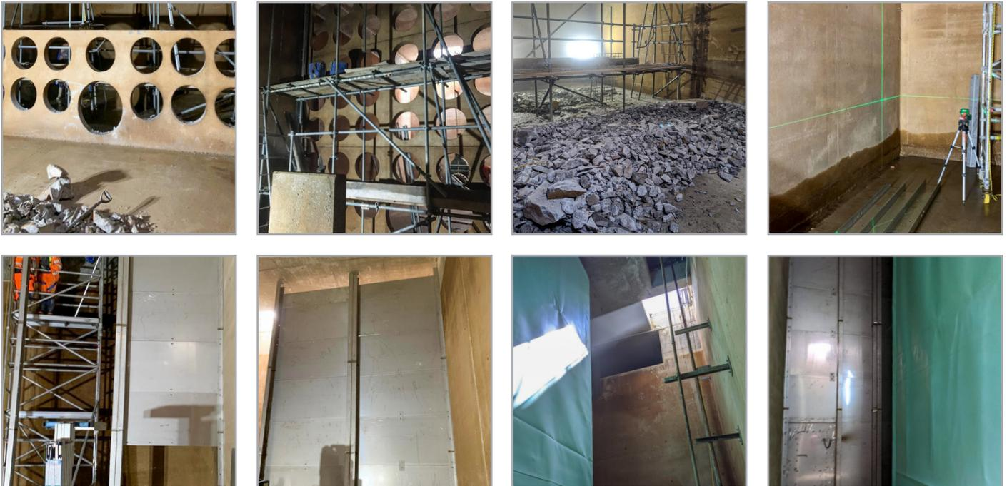
Stonbury was contracted to produce and install a new solution to increase the water quality output from two Water Treatment Works contact tanks, after the client's recent step tests highlighted that at flows exceeding 20MI/d, output failed to meet the minimum disinfection contact requirement.
