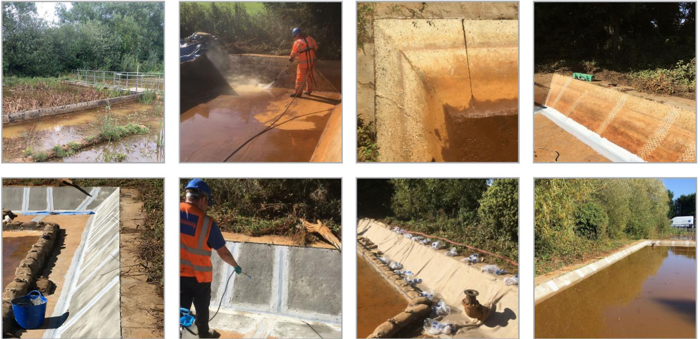
As the main contractor for refurbishment works, a framework client required Stonbury to install a cofferdam system and carry out repairs to a settling tank at a water treatment works.
