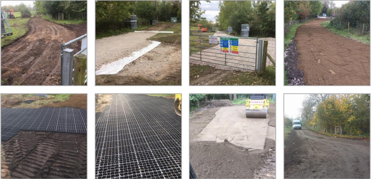
Stonbury was contracted to construct a new trackway to improve access to a pumping station and extend the existing turning area. The works were required as the existing track became unusable during flood events and restricted emergency access to the pumping station.
