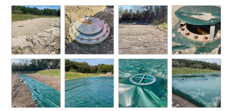
Stonbury attended an emergency response to replace a Start Up To Waste (SUTW) Slurrybag on a wastewater treatment site in the Northwest after the existing bag had failed.
