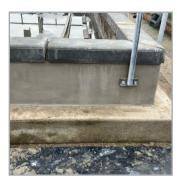
Stonbury's concrete repair work has prolonged the life of a primary settlement tank on a sewage treatment works in the Midlands.
