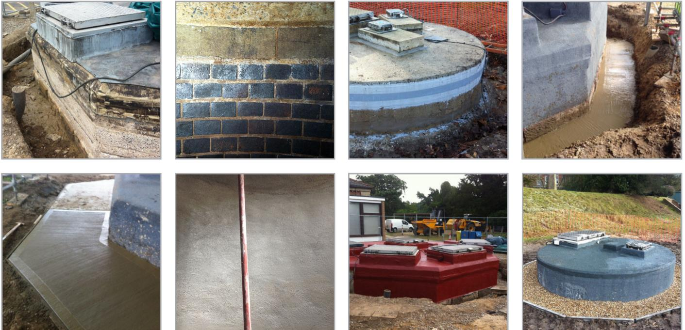
Stonbury were contracted by a framework client to complete ingress repairs to five, 3m deep, slow sand filter wells, at a WTW (Water Treatment Works). One of the wells was a 100 year old structure.
