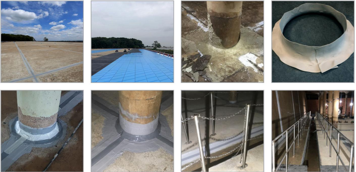
A client approached Stonbury to complete a routine flood test as a part of a flood test and cleaning programme. The flood test was carried out over five days due to the roof's size - approximately 12500M2. The flood test revealed points of ingress and internal coatings that had failed.
