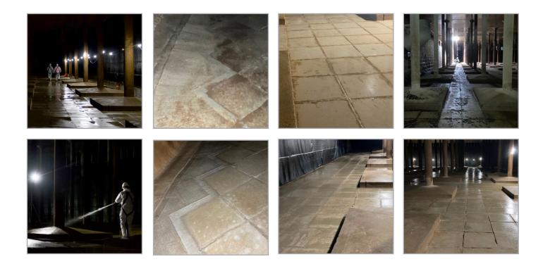
Companies within the Stonbury Group were enlisted to provide a chemical clean and baffle curtain modifications within a treated water reservoir to reduce the potential presence of bacteria and remove dead spots within the tank.
