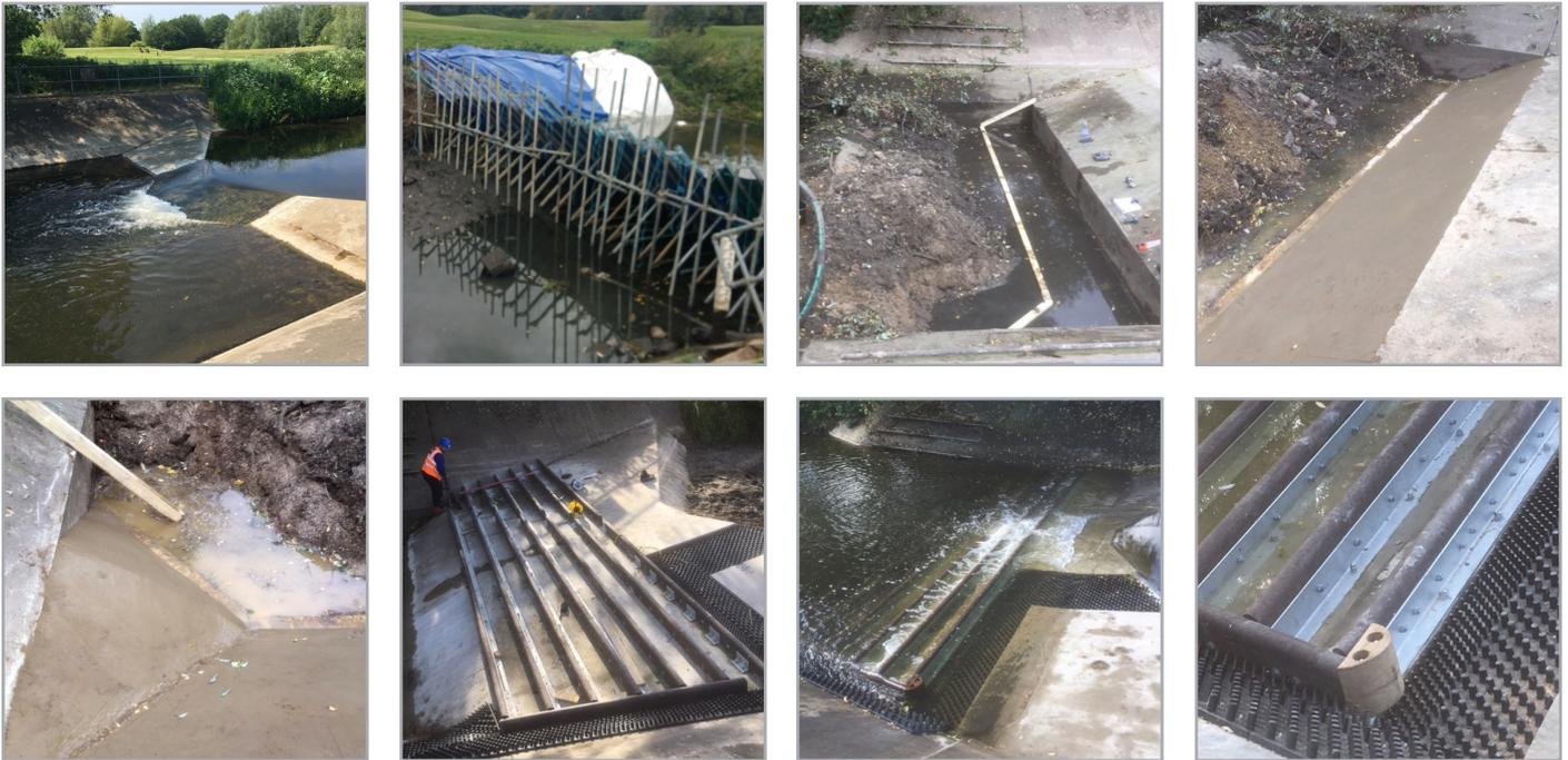
Stonbury were contracted by the Environment Agency to construct a new fish and eel passage on the River Colne, allowing safe migration over an existing gauging weir.
