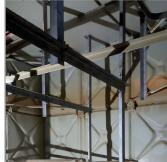
Refurbishments were required on the 0.9 trillion-cubic-metre tank due to degradation of the side panels and instability of the roof. The refurbishments, which have eliminated the requirement for a new tank, have increased the lifespan of the asset by twenty years, saving Stonbury's client over two million pounds.
