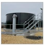
Stonbury delivered a 55m3 sectional steel storm tank on a wastewater treatment site to facilitate compliance with new storm volume regulations.
