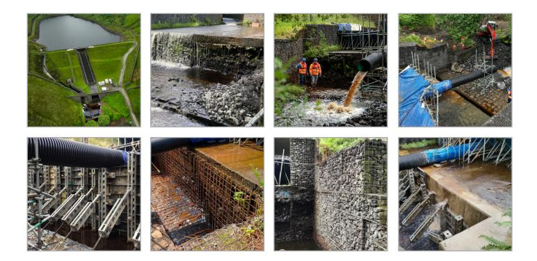
Stonbury was contracted to deliver repairs to a spillway in Lancashire after the existing gabion baskets supporting the structure had degraded.
