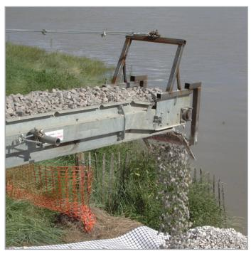
Stonbury was called in by the Environment Agency to solve a challenging problem. A mud flood bank on the River Avon at Pill had slipped, threatening the integrity of residential flats that were situated alongside a stretch of the tidal reach.
