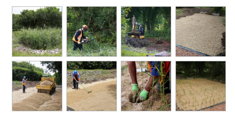
Stonbury were engaged to carry out refurbishment works to a reedbed system at a Water Recycling Centre (WRC) in the South of England. The site serves a small community, with the reedbed providing settlement and treatment capacity for effluent, before it reaches the water course. The works were required as the reedbed had ceased to be effective, due to sludge, overgrown reeds and leaf litter.
