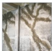
Earlier in the year, we began carrying out repairs to a failing reservoir which showed signs of severe water ingress. The original scope included 180 linear meters of crack repairs. However, following an inspection, this increased to more than 300.
