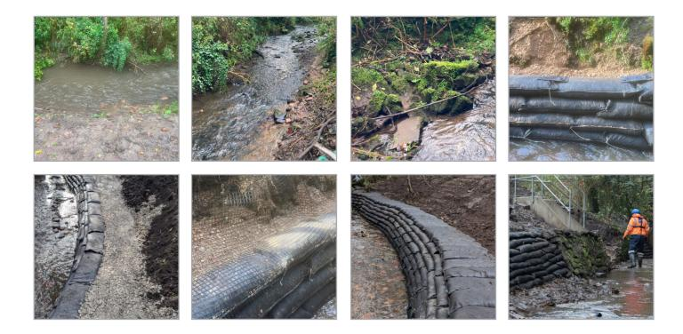
Stonbury delivered a long-lasting hybrid green engineering solution to re-shape and stabilise a section of riverbank after the existing sandstone retaining wall had eroded.
